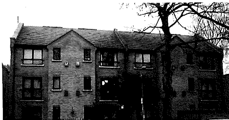
The Cambrian Centre (ground floor) and Caplan Court (top 2 floors)
